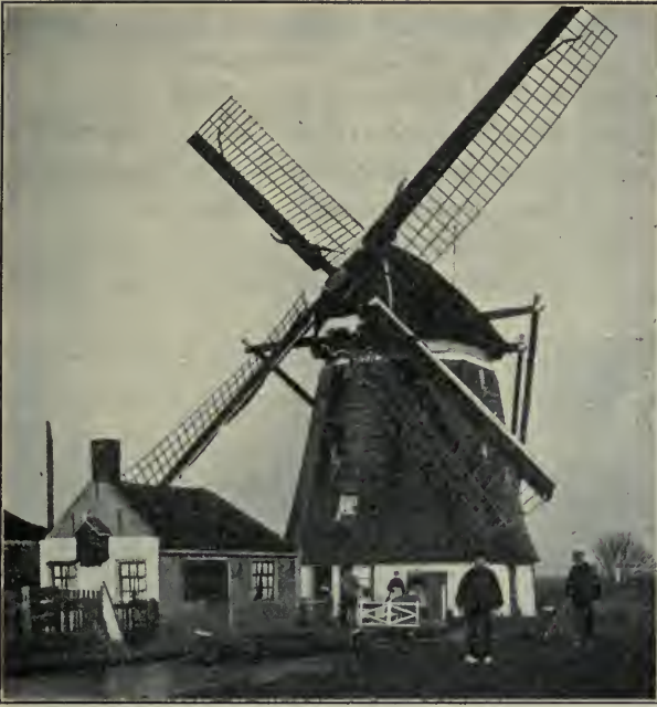
FIG. 540. — A Dutch windmill, used for pumping the water from the low lands behind the dikes.
